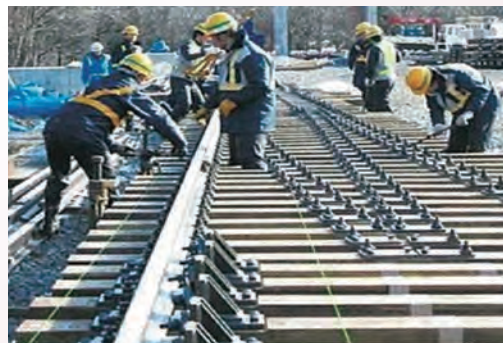
● Practical training with a turnout ●
