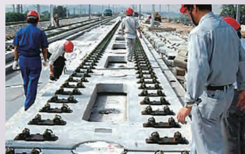
● Slab installation training (People's Republic of China) ●
