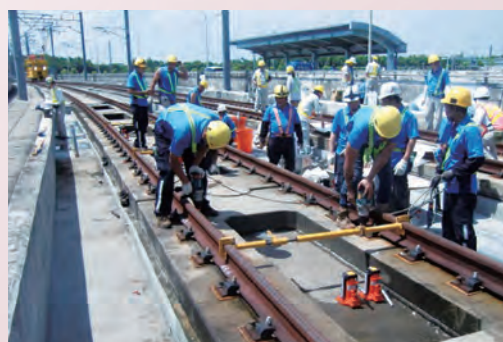
● Practical training with slab tracks (Taiwan High Speed Rail) ●
